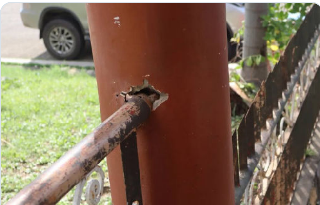
PHOTO 7 · RAILING AND COLUMN
